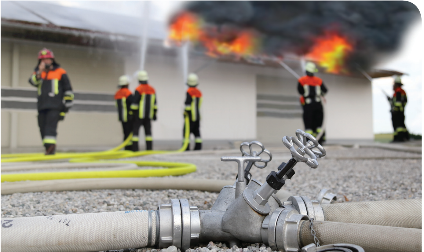
Fire caused by an electrical short circuit or overload resulting in the stoppage of production for more than 24 hours is classed as a dangerous occurrence in the UK
